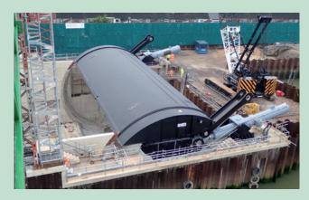
Macrete supplied 24nr precast concrete flood defence units for incorporation into the tidal barrier works. The units were in the shape of an inverted arch and would provide the base for the movable steel tidal barrier once installed.
