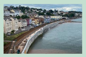
Macrete supplied precast concrete walls and vehicle units to protect the existing railway line from the effects of coastal erosion.
