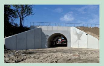
Macrete designed, manufactured, supplied and installed precast concrete abutments, cill beams, both standard and tapered flexi arch units, parapets, capping units, spandrel walls and wing walls.
