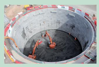
Macrete Ireland Ltd supplied 3.05m, 5.00, 6.00m & 25.00m shaft linings and corresponding cover slabs to the upgrade of the sewer and drainage system around Stroud Gloucestershire. The aim of this scheme is to provide a reliable sewer network and create more storage capacity in times of flood. By doing so, the local river health will also benefit. Materials were supplied to Galliford try on behalf of Severn Trent Water.
