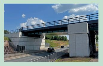
As part of the overall scheme to open a new station at Headbolt Lane, Kirkby, Merseyside and facilitate the laying of additional track Macrete Ireland Ltd supplied precast concrete abutment hollow blocks, wing walls, coping walls and cill beams to the reconstruction of UB55 on behalf of Buckingham Group Contracting & Network Rail.
