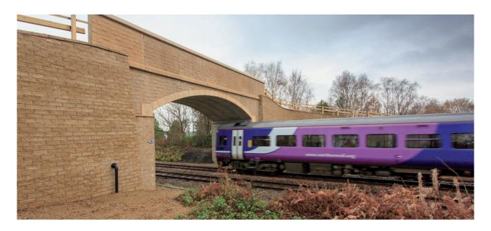
Our ethos of continuous product development and innovation has resulted in the company bringing to market a range of patented technologies such as the flexi arch bridge system, universal shaft linings and the vacuum-flush retention tank system. Since developing the flexi arch (pictured above) we have delivered more than sixty such structures across the UK and Ireland, and the system is also approved for Network Rail implementation.
