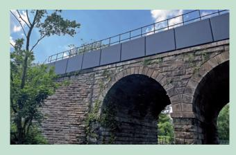
As part of the overall scheme to open a new station at Headbolt Lane, Kirkby, Merseyside and facilitate the laying of additional track Macrete Ireland Ltd supplied precast concrete robust kerbs pigmented black during the casting process to the reconstruction of UB56 on behalf of Buckingham Group Contracting & Network Rail.
