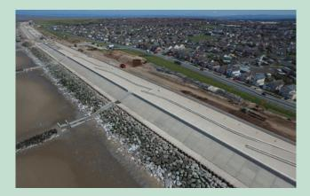
This scheme opened to the public on June 1st, 2018. Since 2015 Macrete had manufactured and supplied over 10,000 precast elements to the works, consisting of revetments, wave walls, steps, stairs and promenade features.
