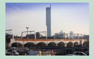
In 2017 Macrete designed, manufactured and delivered precast arches, skewed arches and spandrel arches to this scheme at Manchester Hub.
