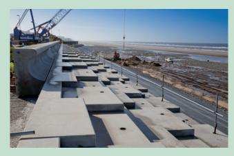
Before the Rossall scheme, Macrete had previously manufactured and supplied over 1,700 precast units to the neighbouring scheme at Anchorsholme on the Fylde coast. A section of coastline was revived by installing revetments, wave walls and stepped wave breaker units. Since entering the coastal defence industry, Macrete have also successfully supplied solutions to schemes at Dymchurch, Redcar and Grimsby.
