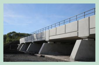
Precast deck units, parapet and edge beams for the refurbishment of Thorndell Viaduct, West Sussex.
