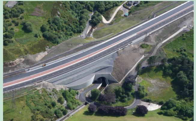
Macrete manufactured and supplied over 17,000m<sup>2</sup> of precast reinforced earth facing panels to the long-term construction of the A465 in North Wales.
