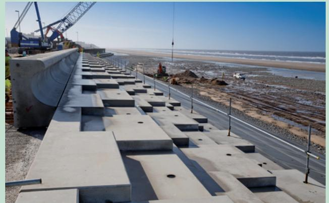
Before the Rossall scheme, Macrete had previously manufactured and supplied over 1,700 precast units to the neighbouring scheme at Anchorsholme on the Fylde coast. A section of coastline was revived by installing revetments, wave walls and stepped wave breaker units. Since entering the coastal defence industry, Macrete have also successfully supplied solutions to schemes at Dymchurch, Redcar and Grimsby.
